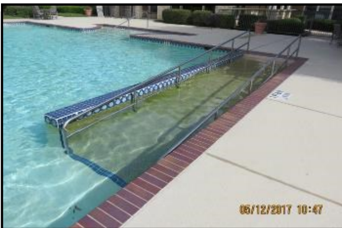
Pool area to rear of leasing office.
