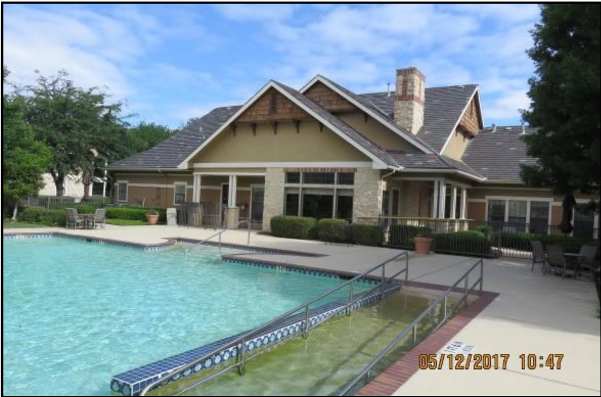
West (rear) elevation of leasing office.
