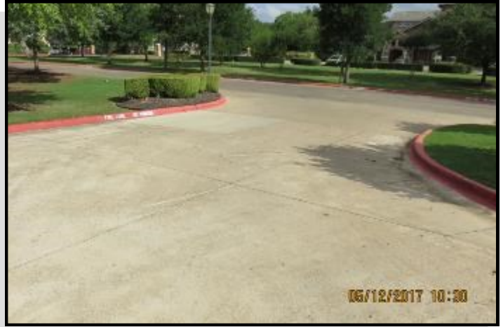
Main entry drive.
