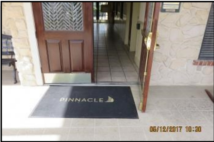
Leasing office main entry.
