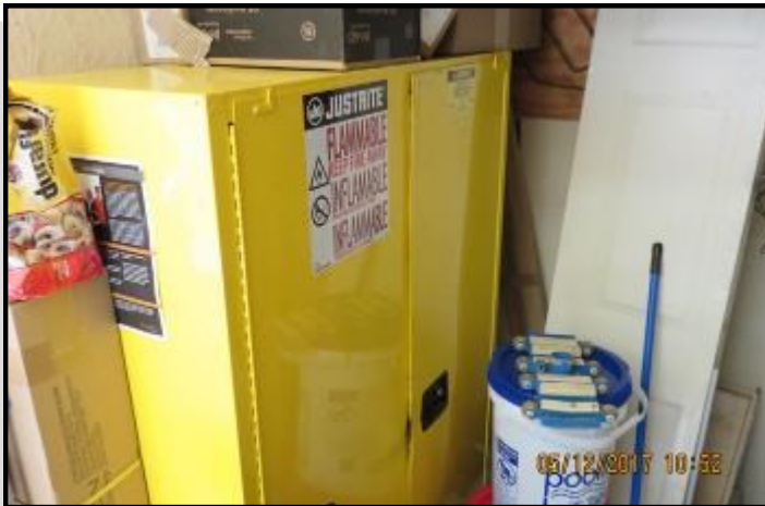
Maintenance supplies stored in a fire proof cabinet.
