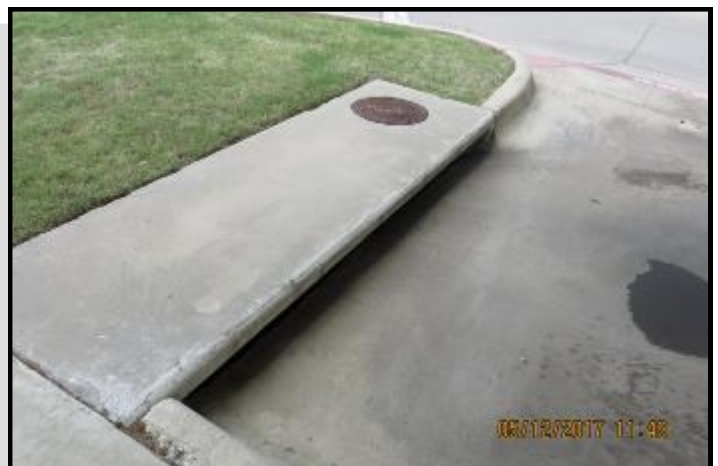
Storm water catch basin.
