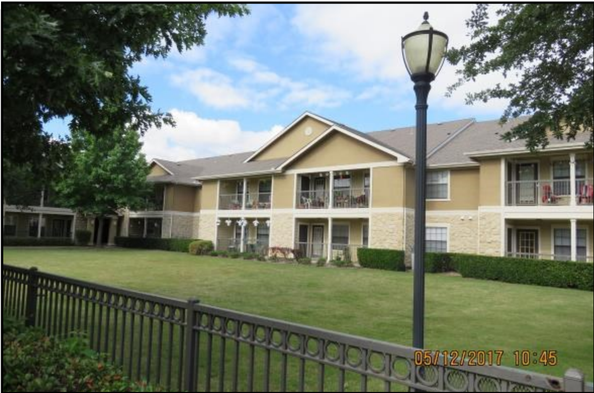
Typical rear elevation of an apartment building.
