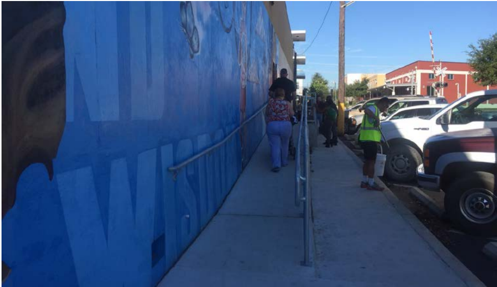
Wheelchair Accessible Ramp to Donation Center/Warehouse
