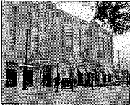
Illustration 2 EXAMPLES OF A TND DEVELOPMENT WITH MULTIPLE-FAMILY USES – COULD DEVELOP IN THE DOWNTOWN VILLAGE AREA OR THE SPECTRUM DISTRICT
