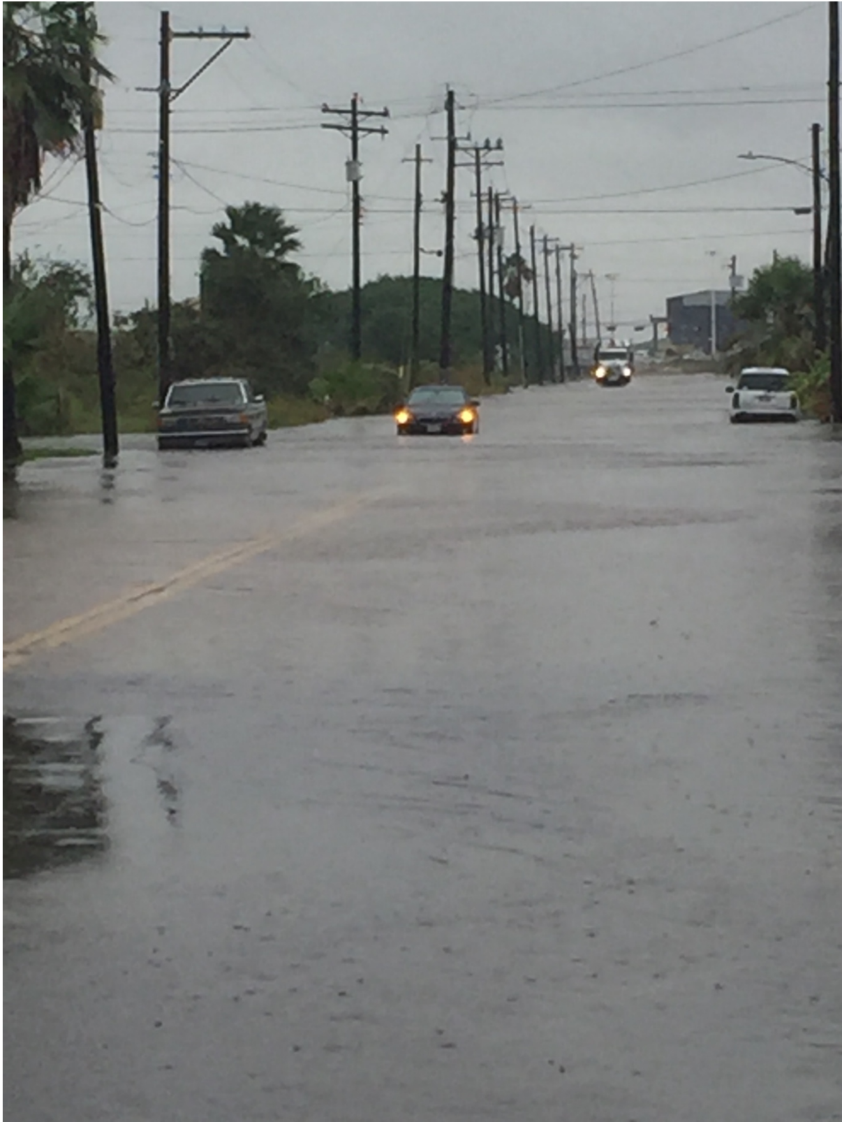
Sandpiper Cove Apartments – Flooding During Heavy Rains
