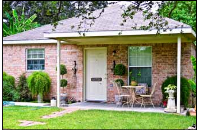
Rural Texans, such as the owners of the newly-constructed home above, have benefited greatly from TDHCA's Homeowner Rehabilitation Program.
