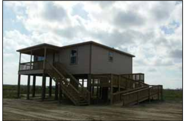
CDBG Disaster Recovery Program's Round 2 rehabilitated, reconstructed and elevated Sabine Pass homes, like the one pictured above, to help low-income Texans weather future storms.
