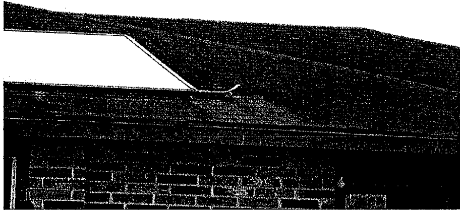
29. View of the roof. Note: The shingles are old and worn.
