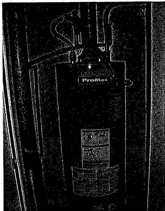
52. View of a typical gas-fired water heater.
