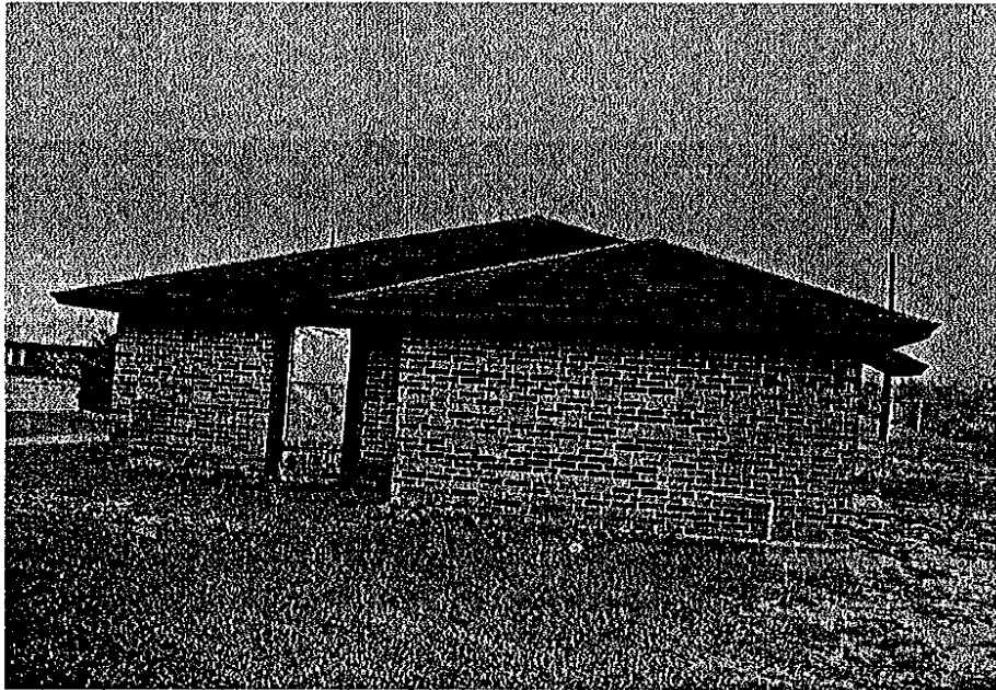
54. View of the side of one of the houses.
