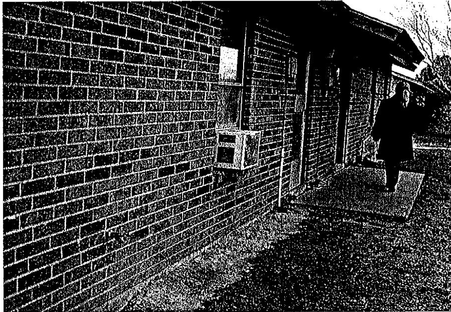
23. View of the rear of one of the houses.
